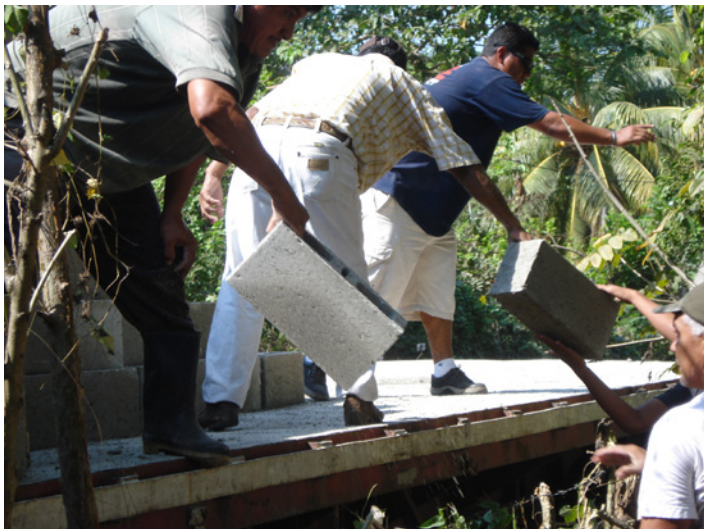
At a central point within the community, family members of 16 beneficiary households in Santa Ana Mixtan unload materials ordered through the voucher catalog. Families used the materials to repair their homes after heavy flooding. Lauren Young/CRS
