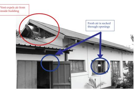
All of these low cost, low maintenance systems are suitable for installation in both permanent and semi-permanent constructions. However, they did present some challenges, including high noise levels created by ducts (solved by installing sound reducers), extractor fans not working correctly, and in some cases, weak public electric systems with insufficient amperage to power the ventilation systems.
