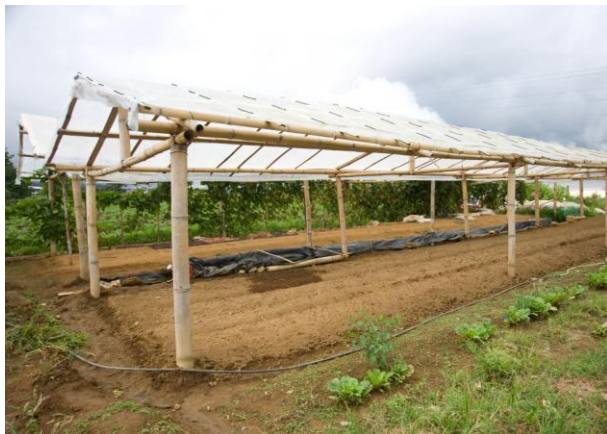
This 100 square meter protective cropping system for vegetables is made of bamboo and plastic sheeting. Each unit costs 13,000 pesos ($289) and lasts more than 3 years. Photo by Dave Snyder.
