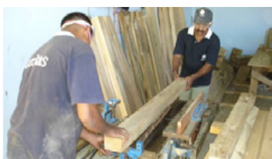
CRS/CSL carpentry workshop cutting timber. Photo credit: CRS/Mehul Savla
