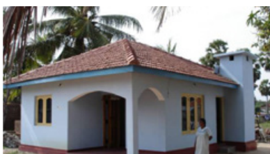
One out of the four different core house designs offered to project participants. They were able to tailor aspects of the house such as colour, door type and so on. Photo credit: CRS/Mehul Savla
