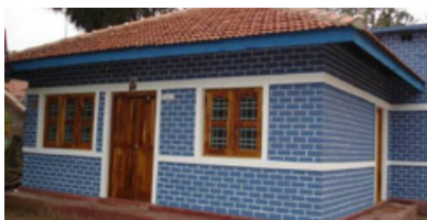
Houses featured disaster resistant features including columns, ring beams, plinths, a sill and a lintel. Photo credit: CRS/Mehul Savla
