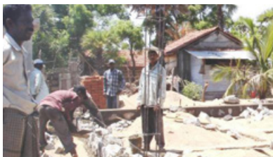
Home owner supervising construction of foundations. Photo credit: CRS/Mehul Savla
