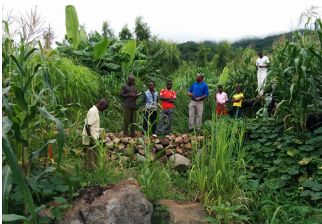
Members of the Watershed Committee standing on a large (about 12-m) check dam, which has reclaimed a barren gully, Lingoni. Photo by Christopher Michael Reichert for CRS.
