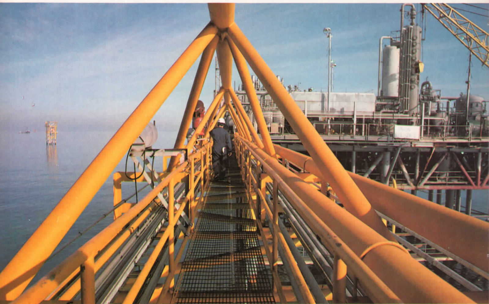
Twenty-six C is two structures in one. One side serves as production center, the other houses control rooms and living quarters.
