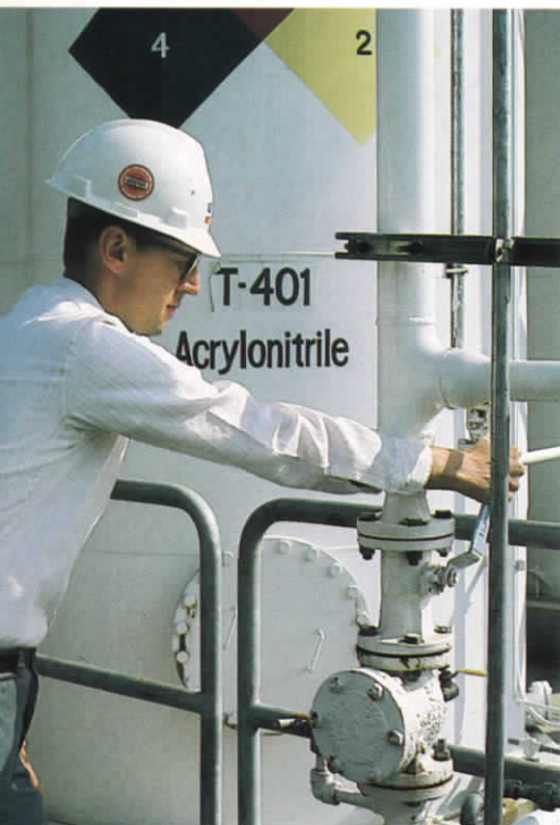
Don Smith, general foreman, says that monomers, the raw materials of polymer emulsions, are stored in five new tanks ranging in capacity from 8,000 to 60,000 gallons.
