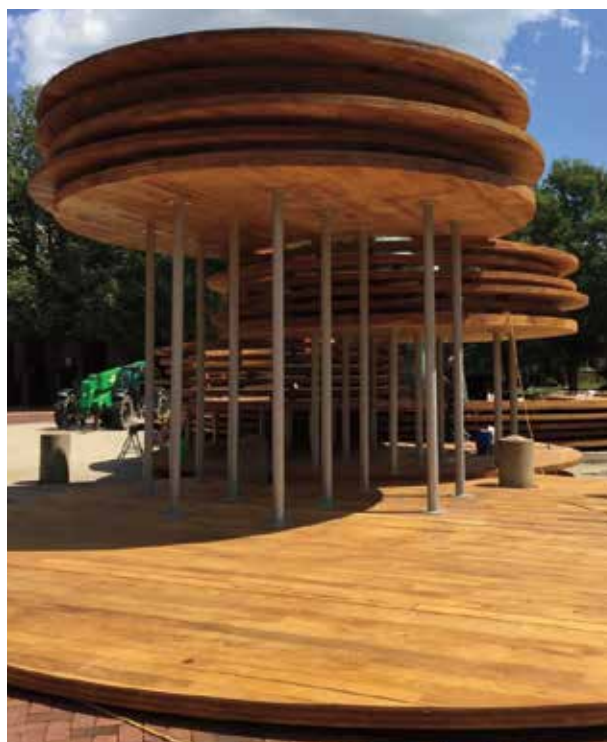
Figure 1. Conversation Plinth - one of the first hardwood Cross Laminated Timber structures temporarily built in Columbus, Indiana. It contained locally sourced hardwood lumber. https://benesonwood.com/portfolio/conversation-plinth/
