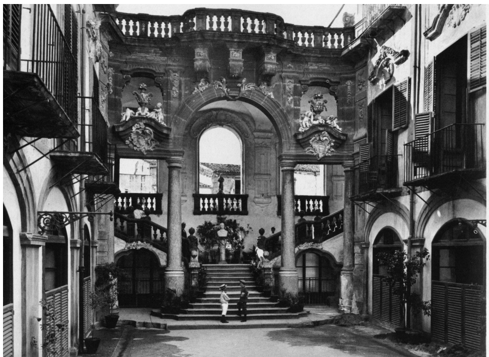
115 (top left) TRAPANI Staircase of the Santuario dell'Annunziata, now the Museo Pepoli, begun in 1639 with decoration added in the 18th century. 116 (top right) PALERMO Court of the Palazzo Cattolica. Probably built about 1720 by Giacomo Amato. 117 (below) PALERMO Staircase of the Palazzo Castel di Mirto, now Bonagia (photographed before the bombing of 1943), said to have been built by Andrea Giganti in the 1750s. Based on Neapolitan models.
