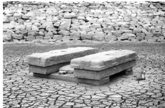
**Water Management and Reservoirs in India and Sri Lanka. Fig. 9** Photo showing the accumulation of an estimated 2–3 m of silt and clay, to near the top of a sluice gate. This reservoir is adjacent to the village of Avinamodugu, south of Vijayanagara (photo by Kathleen D. Morrison).
