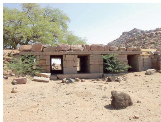
**Water Management and Reservoirs in India and Sri Lanka. Fig. 6** Masonry waste weir, or spillway, to regulate high water levels at the edge of a Middle Period reservoir embankment near the village of Kurugodu (photo by Kathleen D. Morrison).
