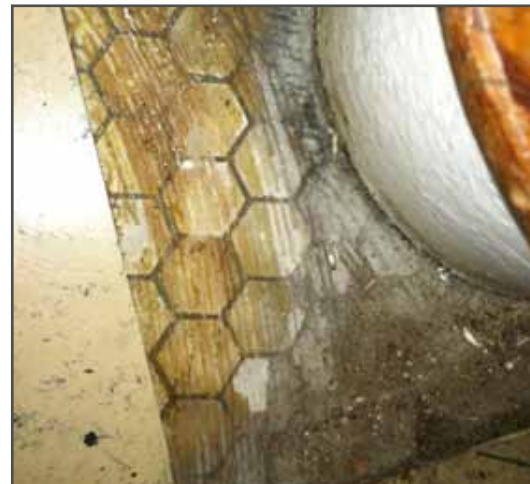
Historic tile found near staircase at entrance, possibly from 1906.
