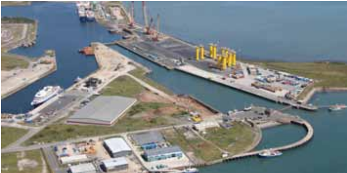
Wind turbine bases, photo courtesy of Furness Enterprises
