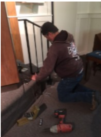
Kenneth Gordon installing the new handrails in the Sanctuary
