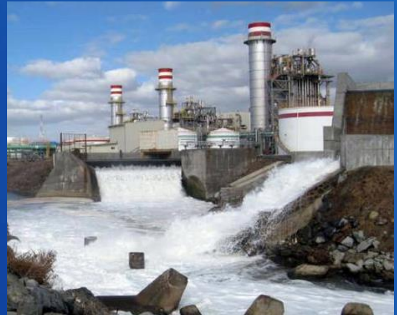
Presidente Juarez power plant at Rosarito Beach
