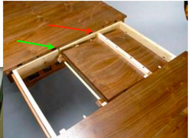
width of the frame narrower than the inside dimension between the skirts by the width required by your ball bearing slides on each side. The normal clearance is 12mm to 13mm (a nominal 1/2") each for most of these slides, but check yours to make sure.
