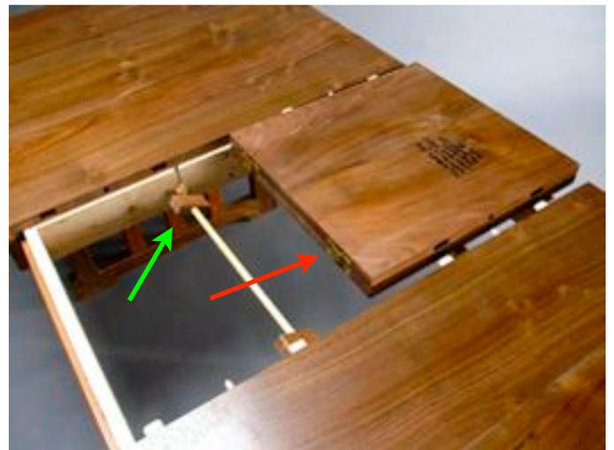
male side (where the tenon is glued in place) the mortises are cut with the narrow tenon width setting. On the female side they are cut with the intermediate tenon width setting.
