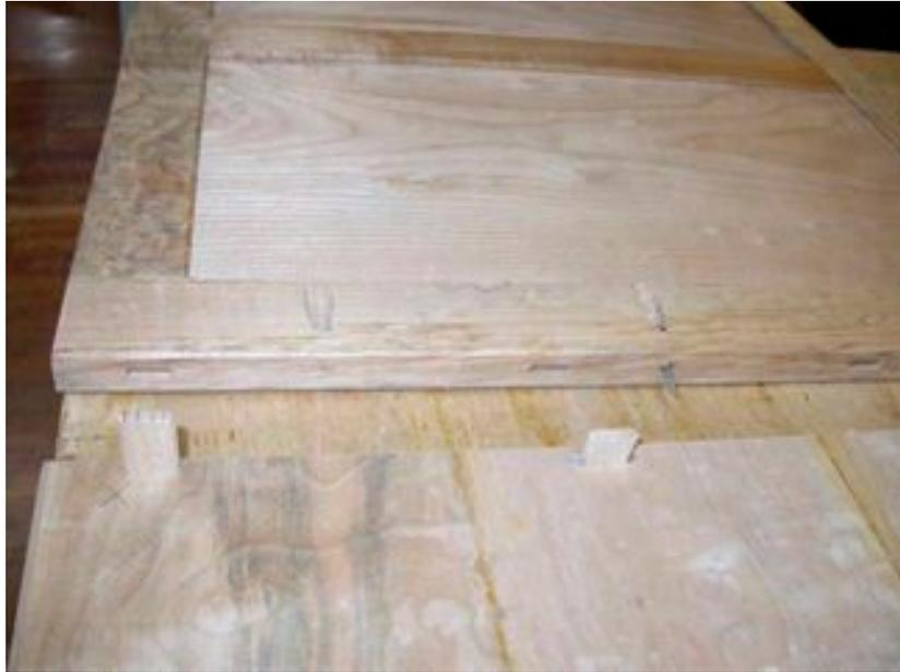
The screw into the tenon prevents the tenon from withdrawing from the unglued mortise in the side stile while it still allows the solid maple pedestal faux drawer
