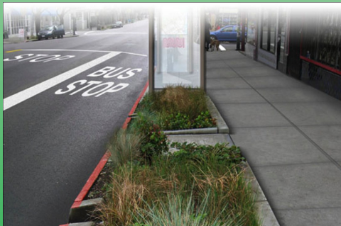
After - Pervious rain garden absorbs and infiltrates the stormwater into the soil.
