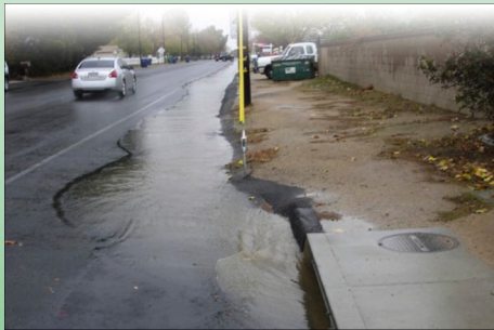
Before - Impervious pavement transporting water into stormdrains after a storm.
