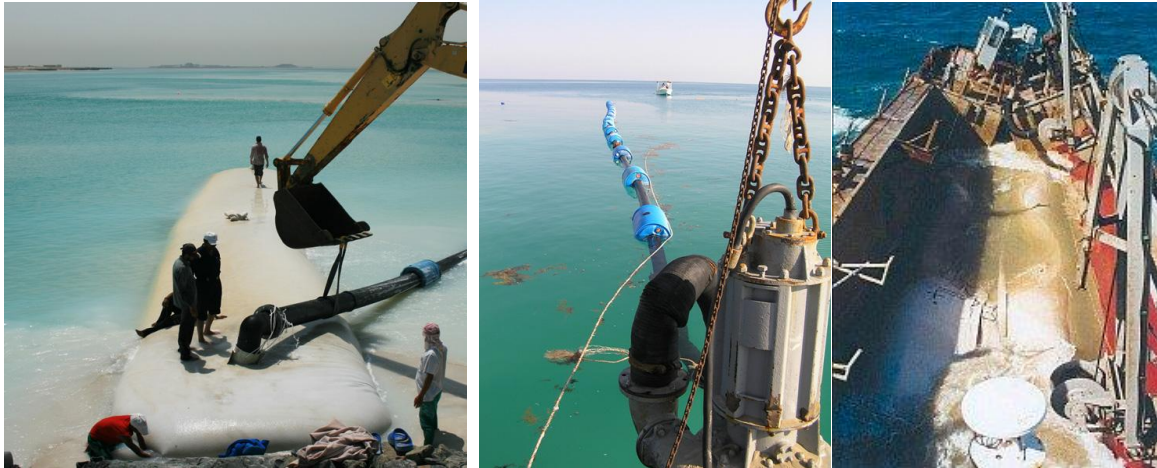
Figure 5 Various construction methods – Filling above water, filling in shallow water with divers, filling in split hull hopper barge and placing in deep water.
