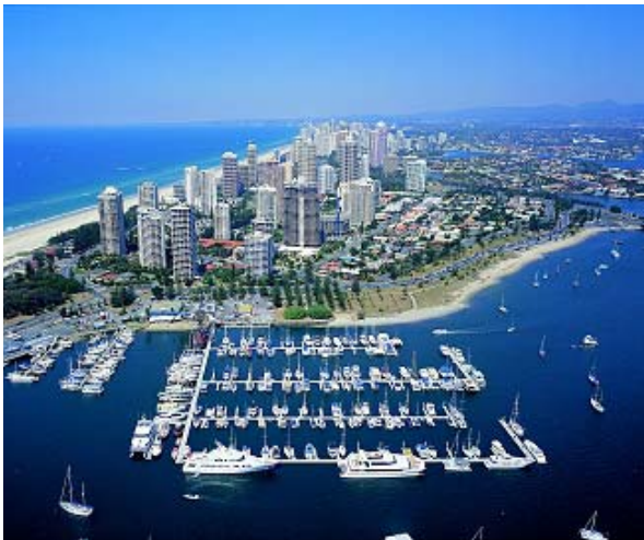
Figure 1 Aerial photo of the Southport Yacht Club marina prior to the extension.
