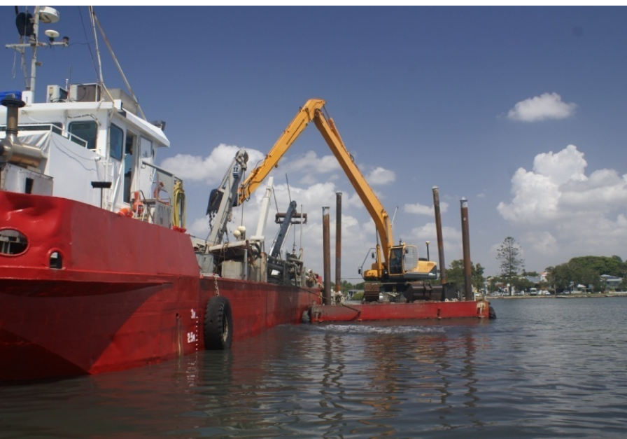
Wynnum Creek Entrance Channel, Moreton Bay Qld
