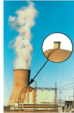
The **vent** on top of the Reactor Building at the Callaway 1000-megawatt pressurized water reactor.
