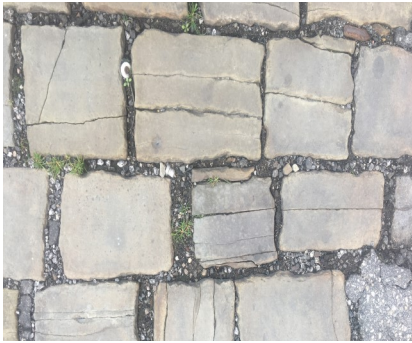
Figure 1. 'Setts' eroding through the modern road surface
